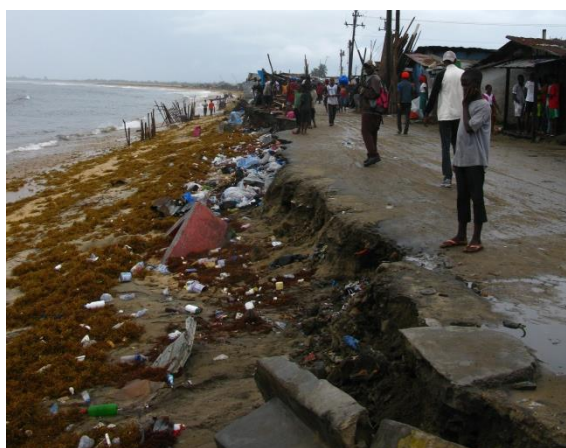
Figure 7: Sea erosion along the coast of West Point (Source: Author, September 2016). Erosion had reached the seaward side road six months after the satellite image in Figure 6 was taken.
